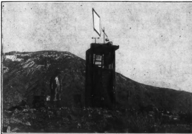
WIND STATION WITH RECORDING APPARATUS FOR DIRECTION AND VELOCITY
