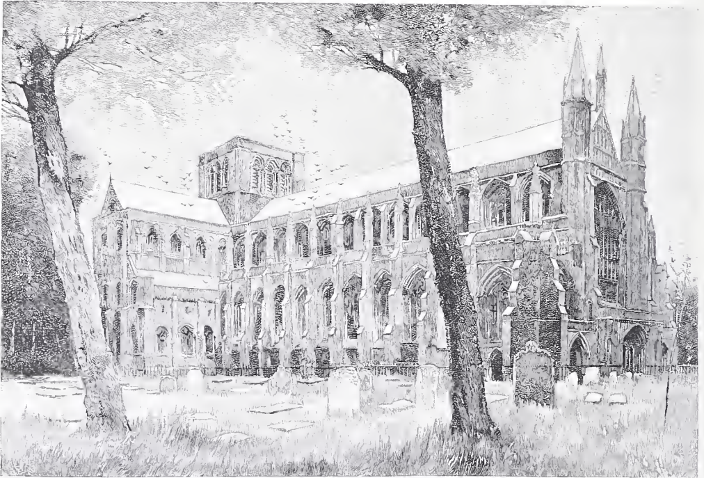
THE NAVE AND TRANSEPT, FROM THE NORTHWEST.
