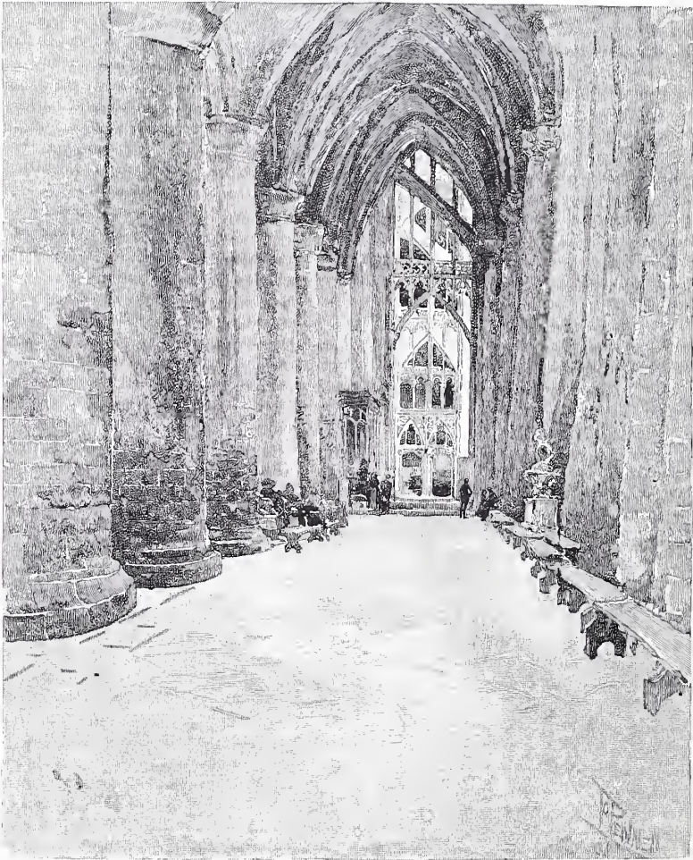
THE SOUTH AISLE OF THE NAVE, LOOKING EAST INTO THE TRANSEPT.
