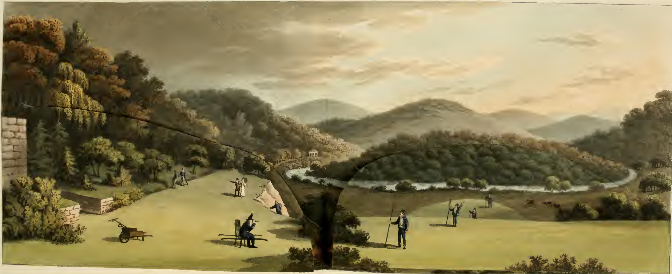
GENERAL VIEW FROM THE SOUTH AND EAST FRONTS OF THE COTTAGE AT ENDSLEIGH, DEVONSHIRE. — DITCHESS OF BEDFORD
