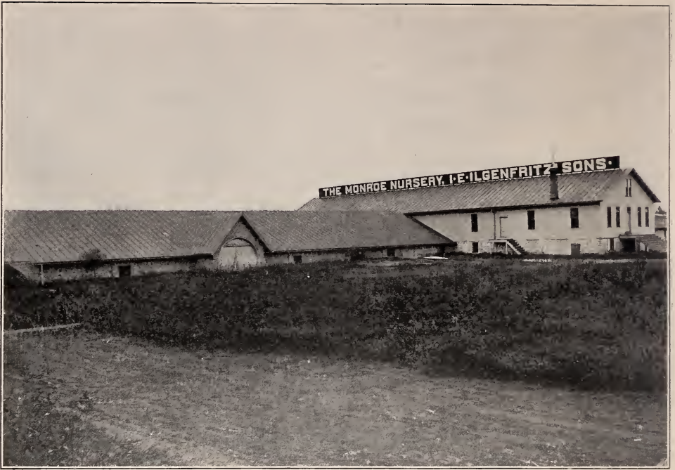
STORAGE CELLARS.—Nos. 1 and 2.
