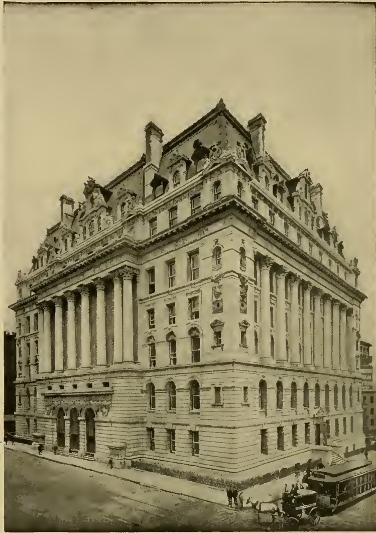
HALL OF RECORDS. Chambers, Reade and Center streets. A splendid fire-proof structure built of steel and Maine granite, for the safe-keeping of real estate deeds, mortgages, etc., of Manhattan Borough, also for Surrogates' Courts and City Offices. Erected 1904, and cost $5,000,000.
