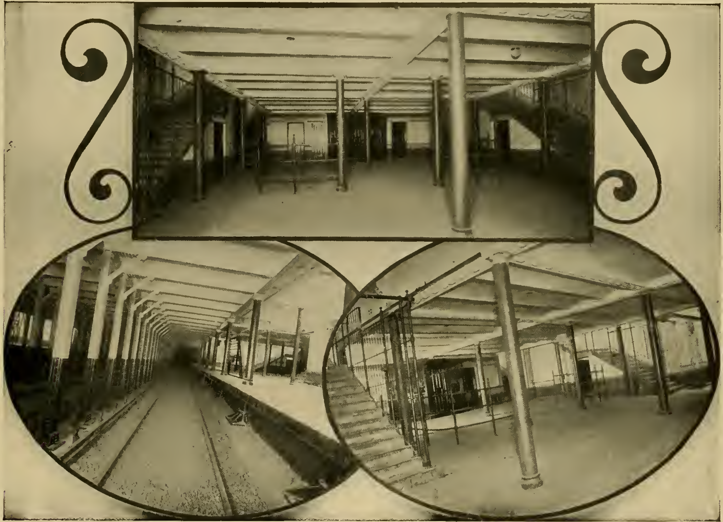
INTERIOR OF SUBWAY. The subway is rectangular, 13 feet high and 25 feet wide for 2-track sections, 50 feet wide for 4-track sections. The bed is of concrete, with steel frame construction, concrete walls and roof, lined with asphalt and roofing felt. It is mostly near the surface, but at certain points drops lower, notably at Columbus Avenue and 104th Street, where the cars pass at a depth of 80 feet. At 169th and 181st street are elevators to stations 110 feet below the surface. The motive power is electricity, using the third rail system. City Hall Park to 96th Street in 13 minutes.
