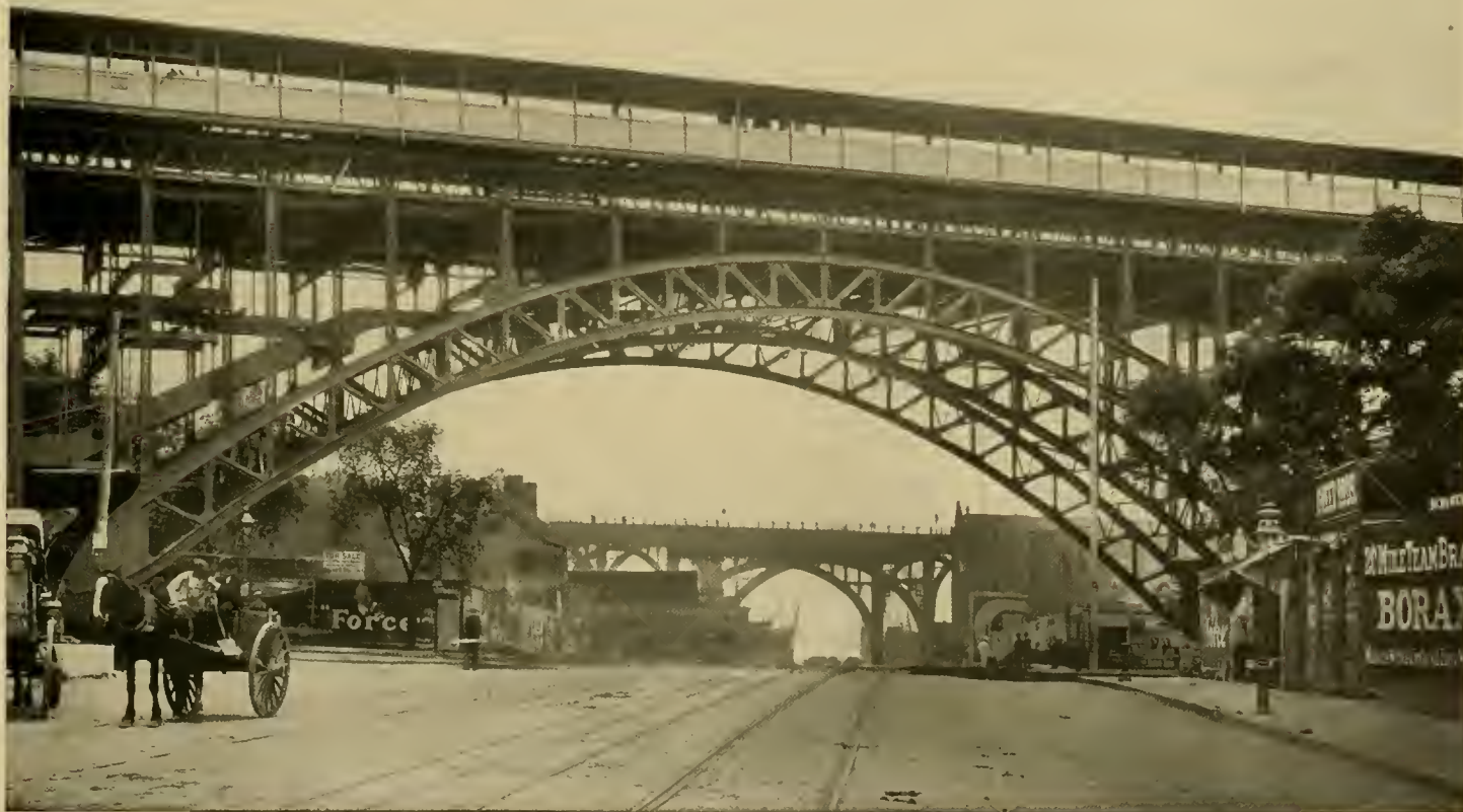
MANHATTAN VIADUCT, Manhattanville. At 125th Street the West Side line of the underground rapid transit system emerges from the subway and crosses the Manhattan valley on a great flying-arch steel viaduct to 135th Street, where it again enters the tunnel, and at 190th Street is more than 100 feet below the surface. The Manhattan Viaduct is a splendid example of American bridgework, and in common with all sections of this greatest engineering feat of the new century, is built to last for all time under the severest strains.
