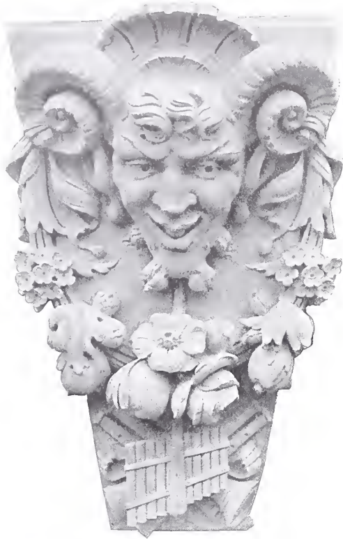
CARVED KEY-BLOCK OVER NICHE IN TERRACE WALL AT DOWNSHIRE HOUSE (see p. 295). DESIGNED BY F. S. CHESTERTON, ARCHITECT
