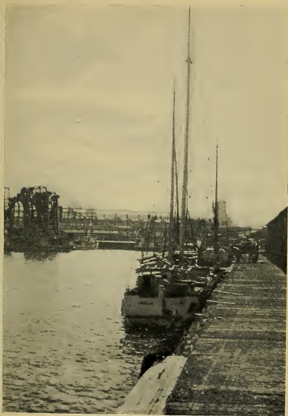
Sailing vessels at the Montreal wharves
