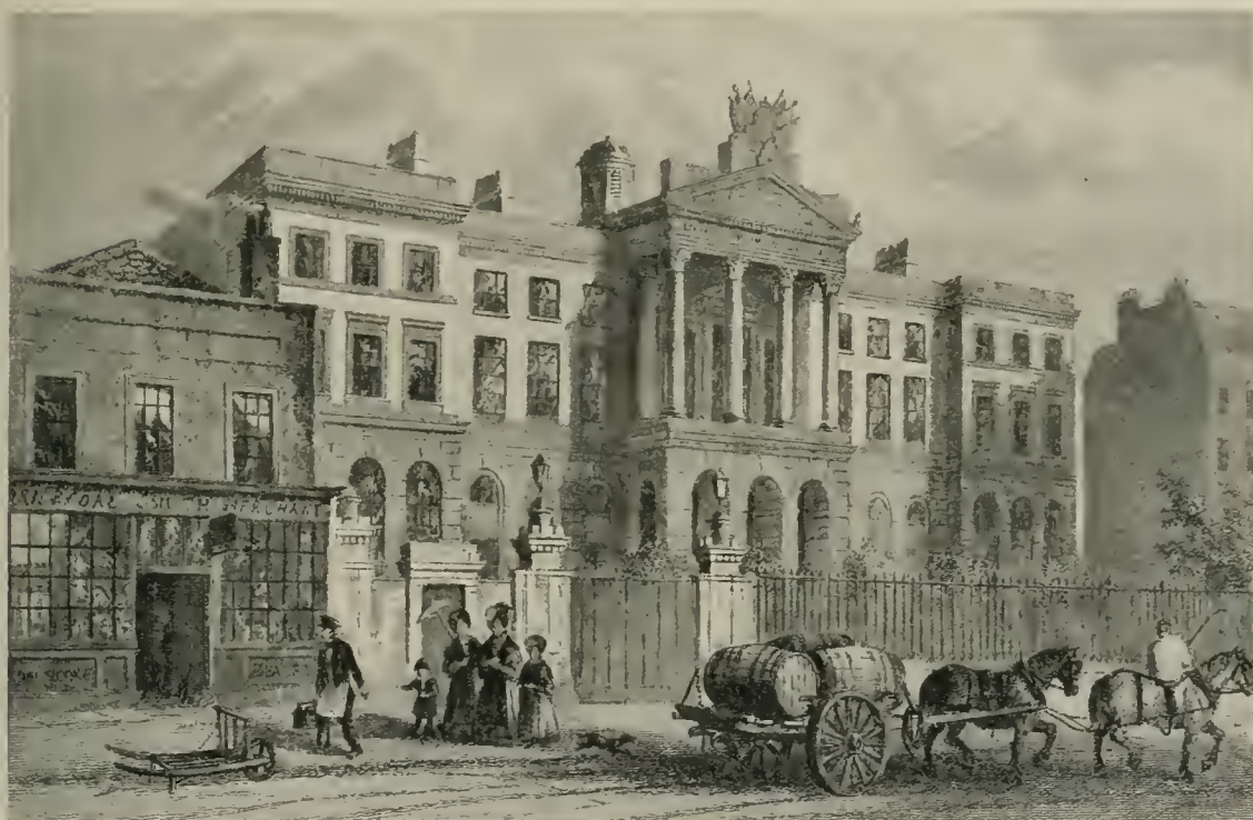
THE LICENSED VICTUALLERS' SCHOOL, KENNINGTON LANE
