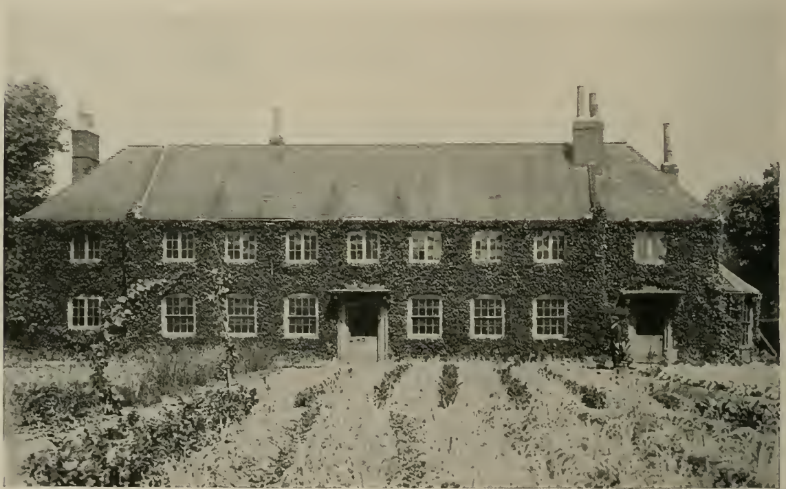
AN OLD BUILDING IN THE GROUNDS OF SAYES COURT, DEPTFORD, WHICH BELONGED TO JOHN EVELYN
