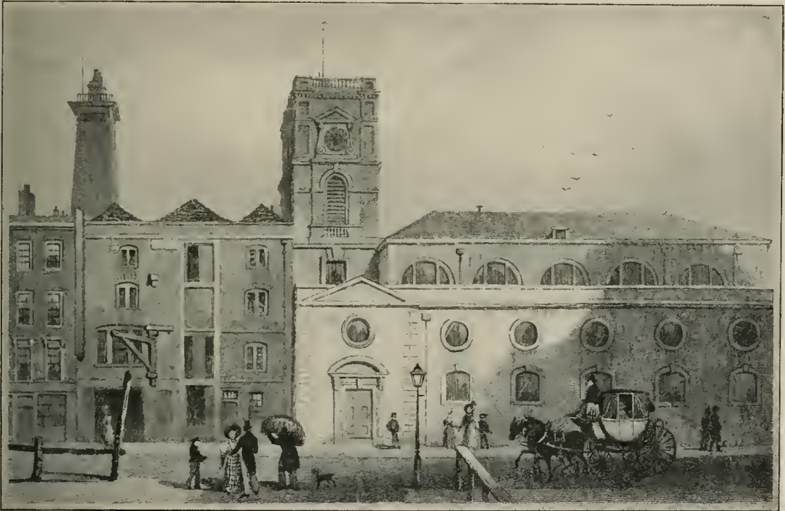
ST. OLAVE'S CHURCH IN TOOLEY STREET, SOUTHWARK, AS IT APPEARED EARLY IN THE NINETEENTH CENTURY
