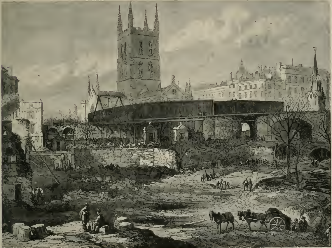
PART OF THE SITE OF ST. THOMAS'S HOSPITAL AT SOUTHWARK BEING CLEARED FOR RAILWAY PURPOSES
