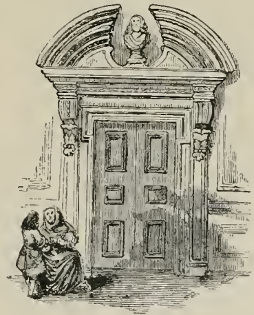
A DOOR IN BOWYER HOUSE
