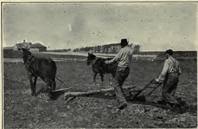
Fig. 61. Filling the ditch with a plow.
