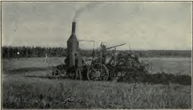
Fig. 54. A tile ditching machine at work.
