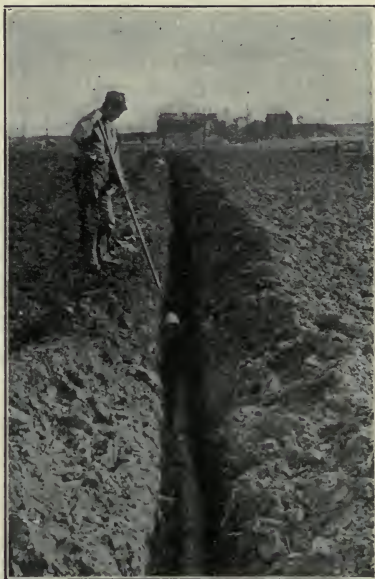
Fig. 59. Laying tile with the tile hook.
