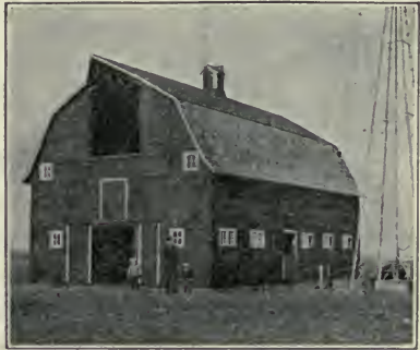
Fig. 285. A general farm barn with gambrel roof.
