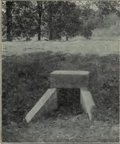
Fig. 97. Concrete culvert after the plan of Fig. 96.
