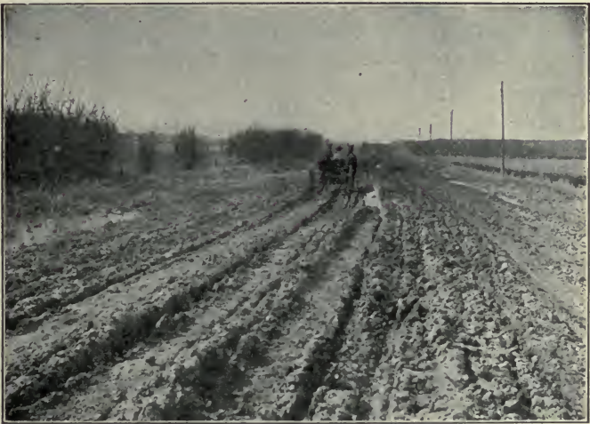
Fig. 81. A typical condition of an earth road on which the drag has not been used.
