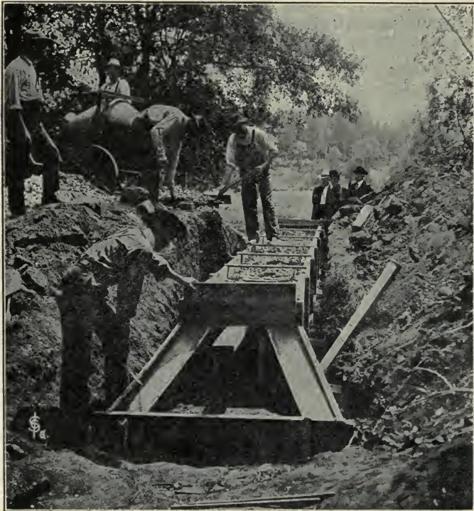
Fig. 95. Making a concrete culvert.
