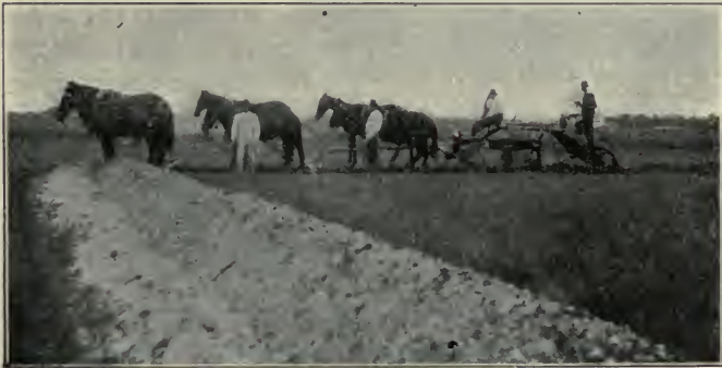
Fig. 62. Filling the ditch with a road grader.
