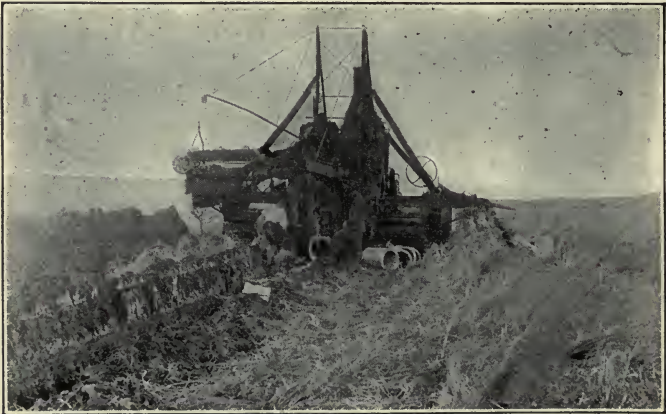
Fig. 55. A large tile ditching machine at work.
