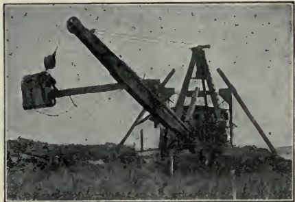
Fig. 66. A floating dredge for digging open ditches.
