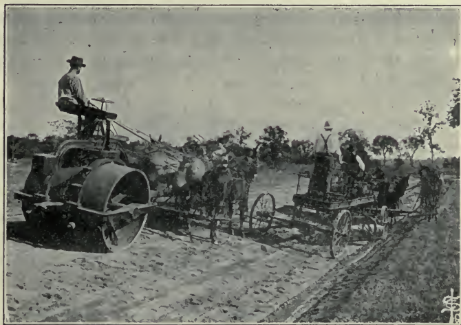
Fig. 91. A scraping grader and a horse roller at work.
