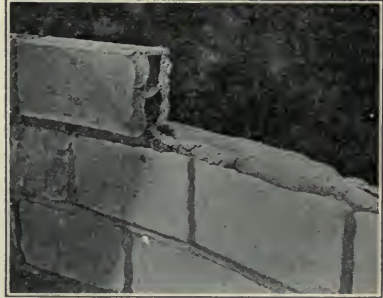
Fig. 297. The wall of the Iowa silo.
