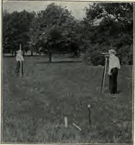
Fig. 50. Taking levels in making a survey.
