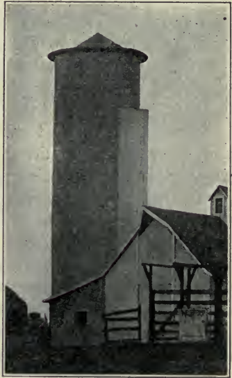
Fig. 304. An Iowa silo with a masonry water supply tank on top.
