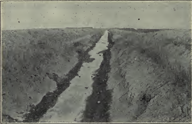
Fig. 43. An open drain.
