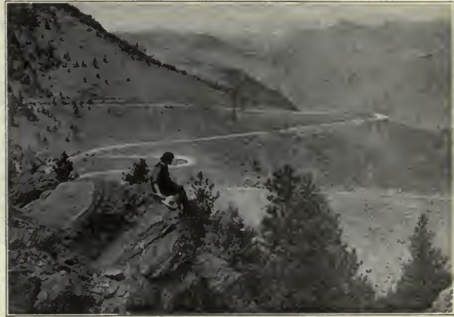
The Auto Road through Denver's Mountain Parks
