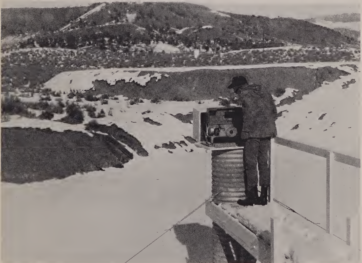
FIGURE 1.—Water-stage recorder installed in reservoir for measuring runoff.
