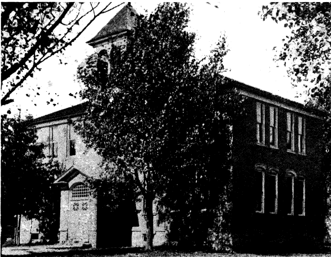
MIDDLETON SCHOOL BUILDING.
