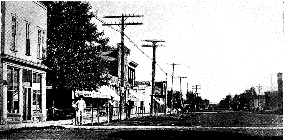
STERLING STREET, LOOKING NORTH.
