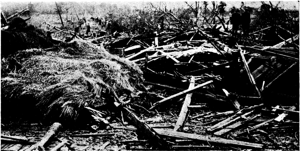
WRECKAGE OF BOWMAN BUILDING—MRS. BOWMAN WAS KILLED.
