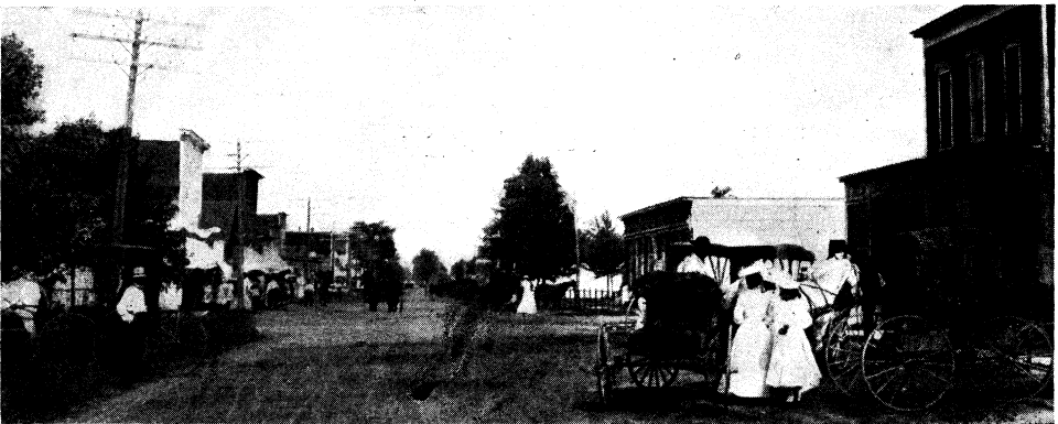
MAIN STREET, LOOKING EAST.
