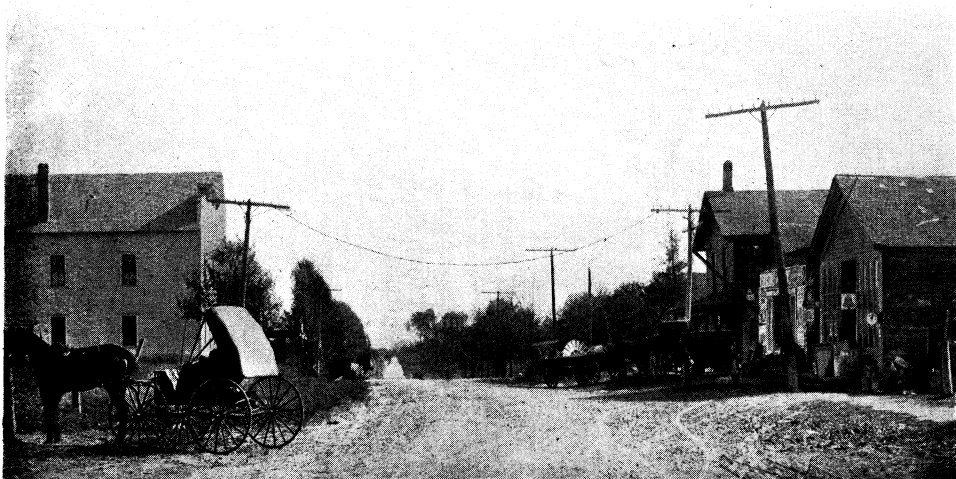
MAIN STREET, LOOKING EAST.
