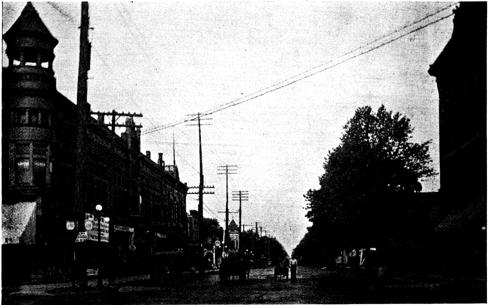
SUPERIOR STREET, 1913—LOOKING WEST FROM STATE STREET.
