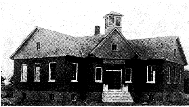
WHEELER'S SCHOOL BUILDING.
