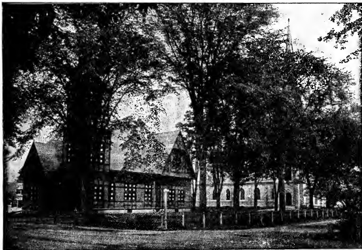
THE SOUTH PARISH CONGREGATIONAL CHURCH, AUGUSTA, ME.
