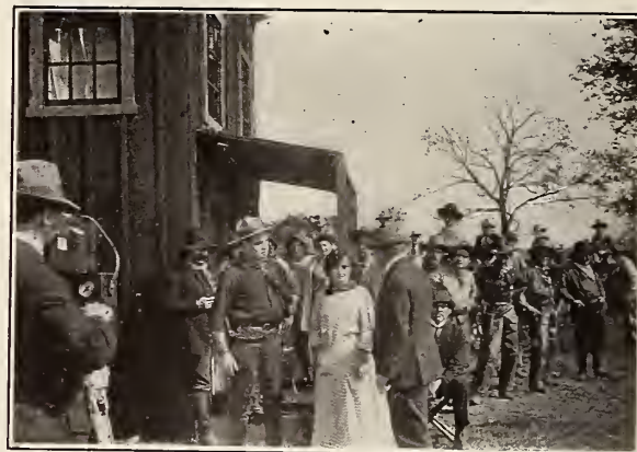
House built by F. J. Grandon, one of the Lubin directors, to be burned down for a photo-play. The people in the picture are the members of the company who played the rôles of the rescuers and rescued. The house was a heap of ashes in less than 30 minutes. The scene was taken on Siegmund Lubin's Betzwood estate.
