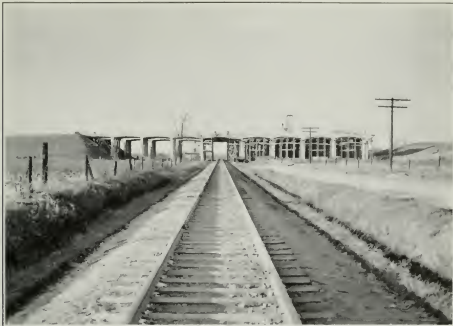
Queen Elizabeth Way — Grade Separation, C. P. R. Crossing near Kipling Avenue
