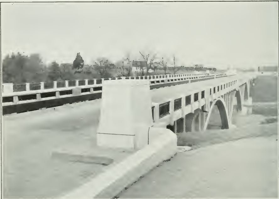
Queen Elizabeth Way — Henley Bridge
