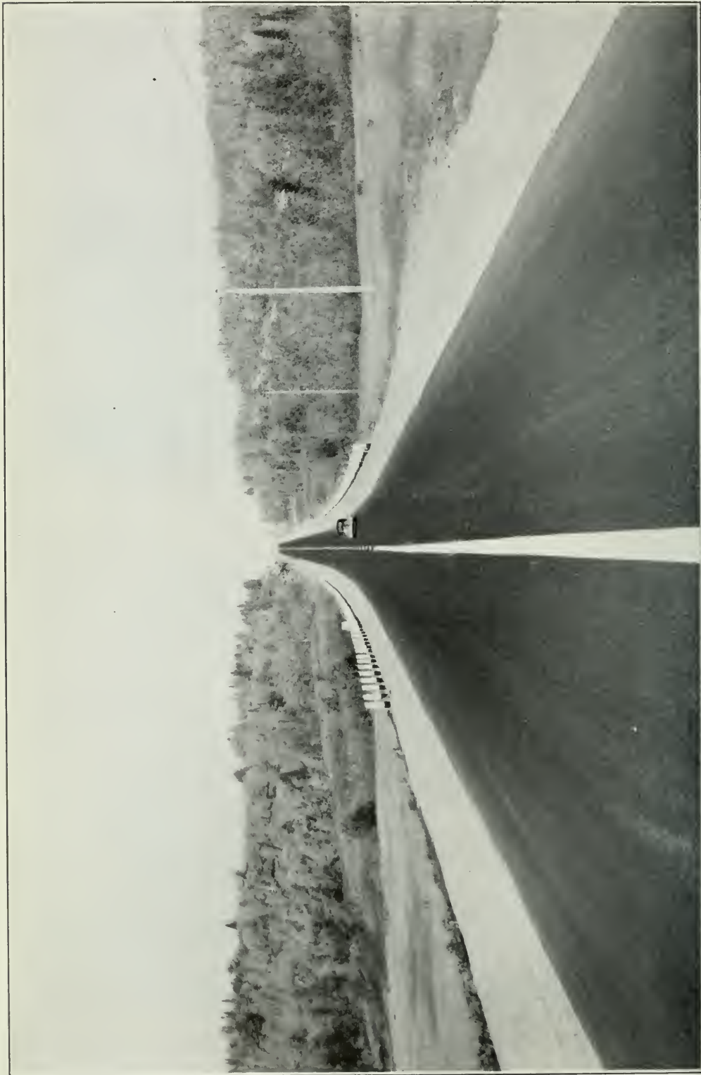
MIXED MACADAM PAVEMENT — HIGHWAY No. 11, NORTH OF NORTH BAY
