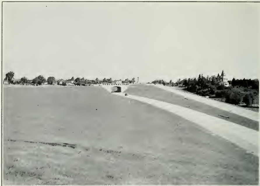
Daylight View — Junction of Highways Nos. 2 and 5 at Scarborough
