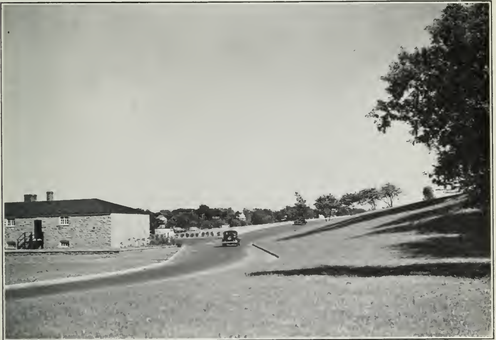
Navy Hall showing new roadway
