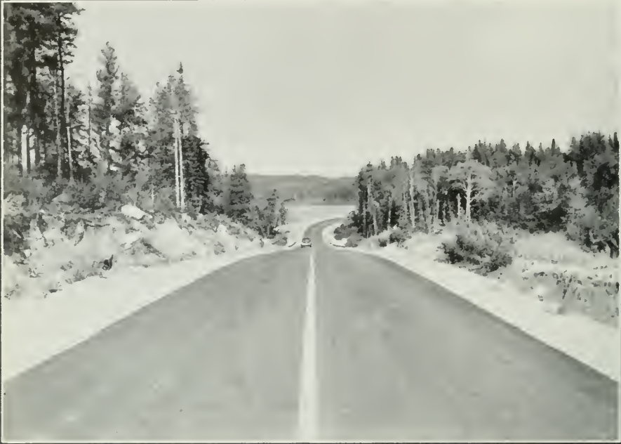
Mixed Macadam Pavement — Highway No. 17, West of Kenora
