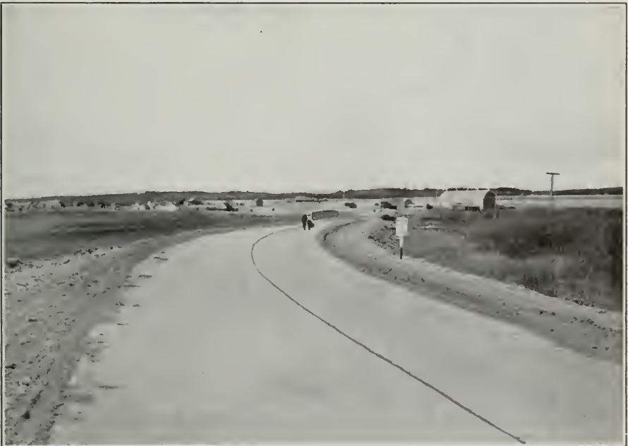
Concrete Pavement, Highway No. 67 at Porcupine
