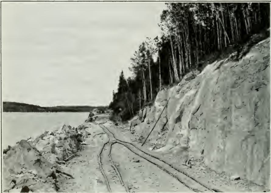
Grading, Nipigon-Geraldton Highway — Rock Cut at Helen Lake
