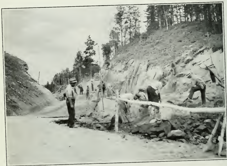
Grading, Highway No. 70 — Rock Cut, North of Nestor Falls
