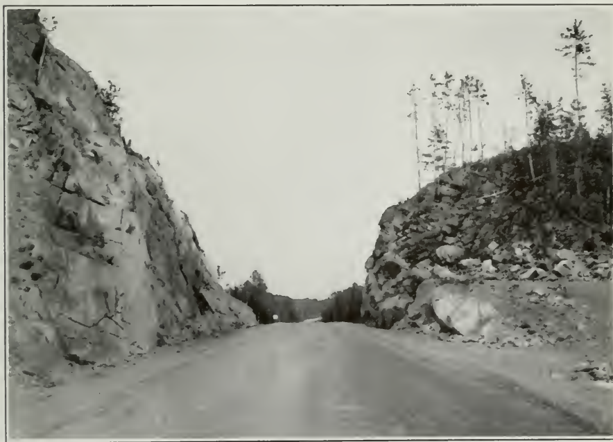
Grading, Highway No. 70 — Rock Cut, North of Nestor Falls
