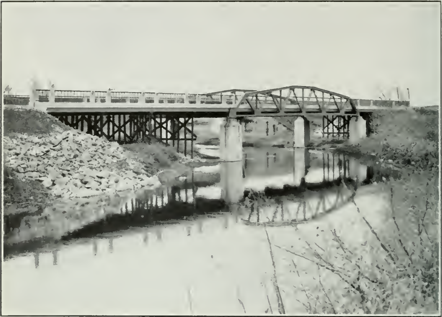
Lost River Bridge, Highway No. 11, North of Kapuskasing
