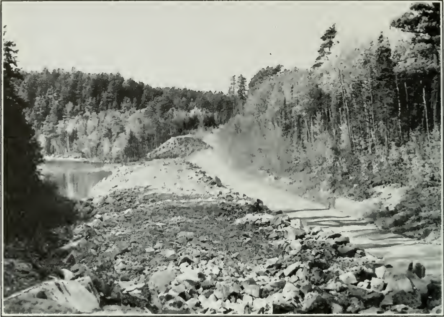
Grading, Highway No. 11 — Fill at Herridge Lake, Timagami Park
