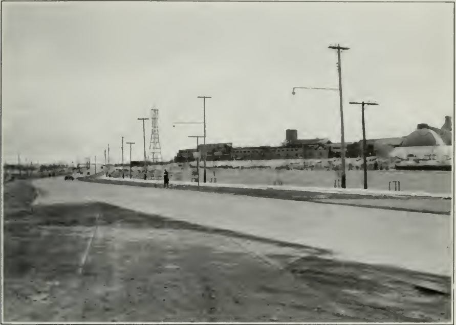
Concrete Pavement, Highway No. 67 at Timmins
