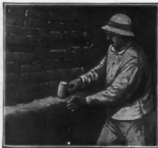
Showing care with which Plibrico is laid in place.
