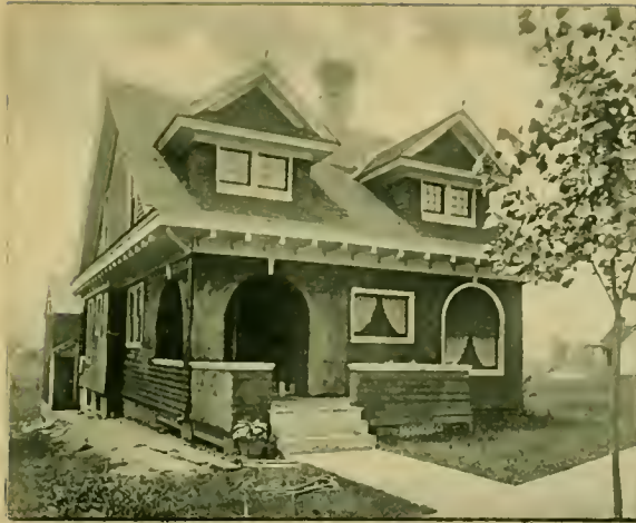
RESIDENCE OF D L WEBB.
