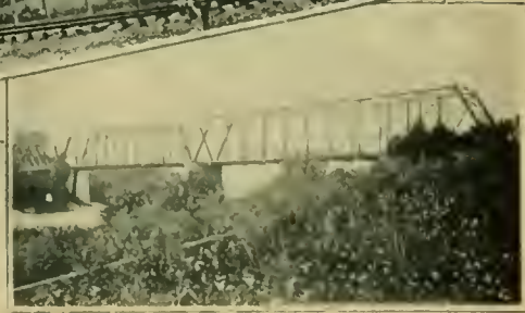
New Bridge over Scioto River.
