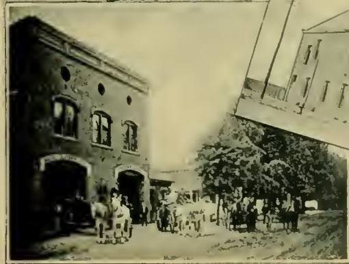
Seventh Street Fire Department.
