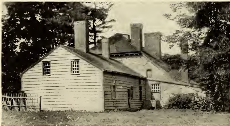
THE EAST END OF THE HOUSE.
