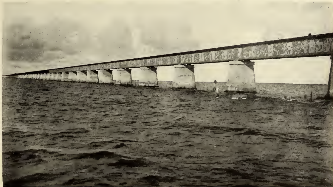
A STRETCH OF STEEL BRIDGE AND CONCRETE PIER CONSTRUCTION.
