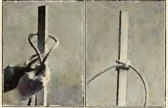
6. HOW TO HITCH A LINE TO A POST.
