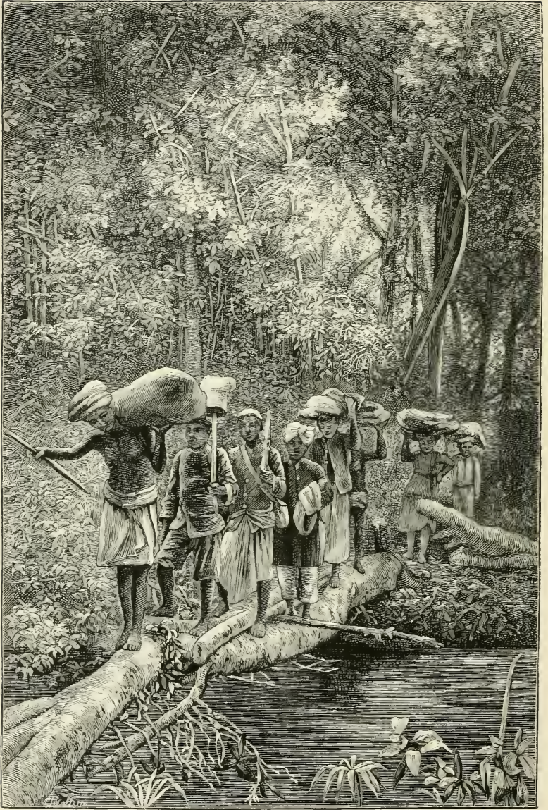
BRIDGE OVER THE MALANGA RIVER.
