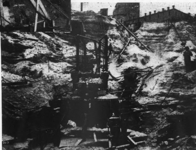
Pumping Sand with the “Return-Air” System in the Quarry of the United States Silica Co., Ottawa, Ill. This illustration shows the tank end of the system which is usually submerged when pumping liquids.
