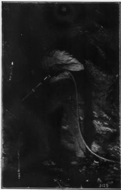
Trimming walls with The "Little Jap"
