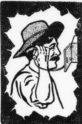
In the shaft.
