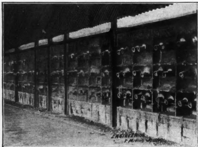
FIG. 3. FURNACE AT WORK WITH FUME NOZZLES ATTACHED
