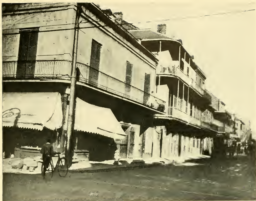
A Typical Corner.
