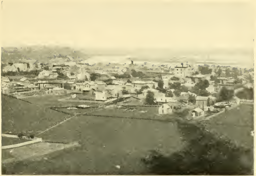
Saint Paul, Looking Southwest. From a photograph taken in 1872.
