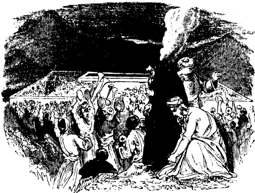
LAYING FOUNDATION OF SECOND TEMPLE.
