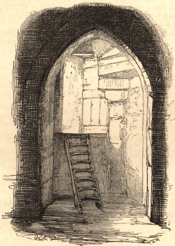
SECRET STAIRCASE IN THE SALT TOWER.
