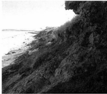
Looking northeast towards Teller. The sunny day made capturing a good photograph in the shadows difficult. The overhanging top of the land can be seen in the upper right. Clumps of topsoil from the upper slumping zone are present down on the beach.
