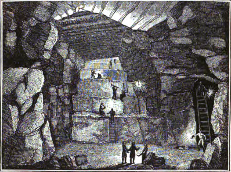
931. A general view of mining operations.
