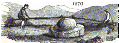
Fig. 1270. represents the rude grinding apparatus used at the lavaderos , or gold washings, in Chile. The streamlet of water conveyed to the hut of the gold washer, is received upon
