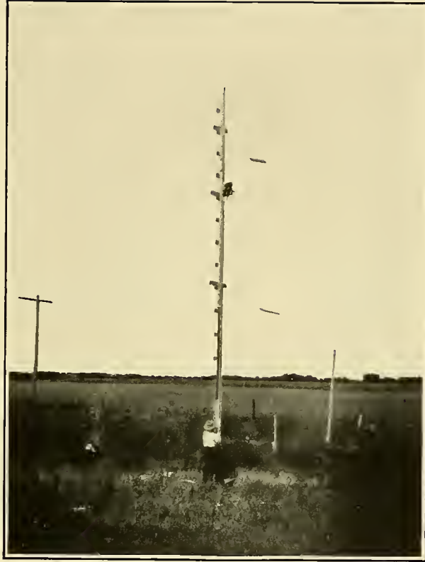
STRUCTURE FOR ELEVATING SIGNAL LAMP OVER TRIANGULATION STATION USED AS MARK.
