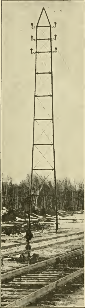
Fig. 175. Steel Tower with Insulators Mounted One above the Other
