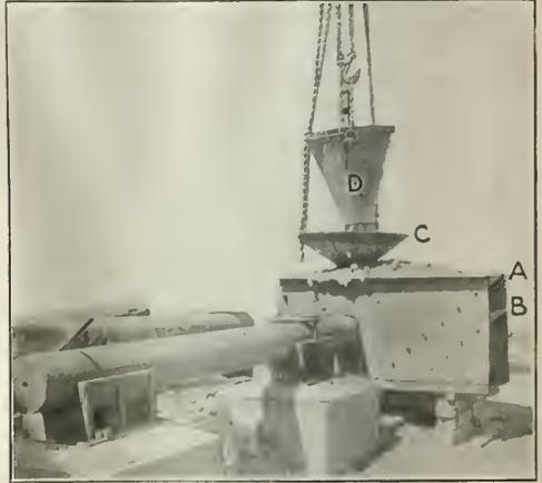
FIG. 2. READY TO IGNITE THE CHARGE OF THERMIT
