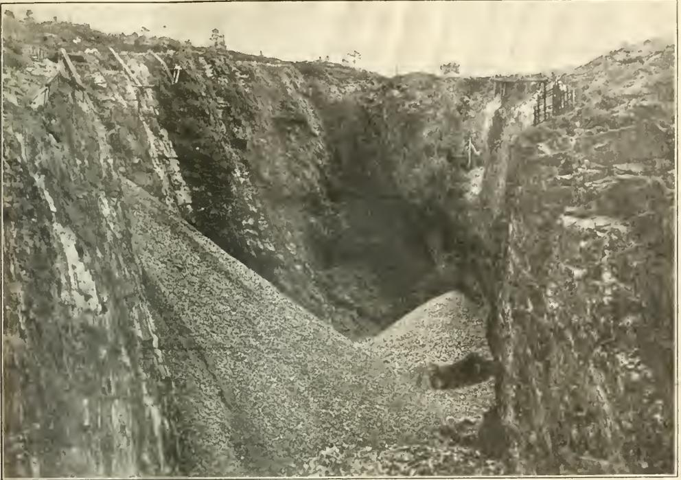
OPEN CUT AT THE CAPTEN MINE. ORE IS MILLED AND HOISTED BY SHAFT
