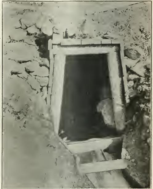
FIG. 4. MEASURING WEIR AND DRAINAGE ADIT
