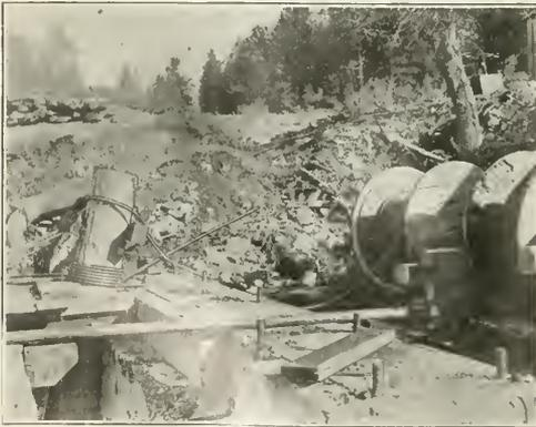
FIG. 3. WIRE-ROPE ANCHORAGES FOR TAKING UP WEIGHT OF AIR LIFT PIPE
