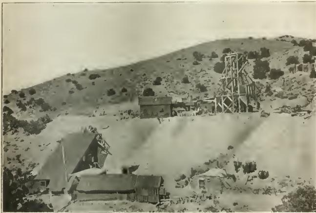
SIMON SILVER-LEAD MINE, MINA, NEV., SHOWING SHAFT EQUIPMENT AND EXPERIMENTAL FLOTATION PLANT
