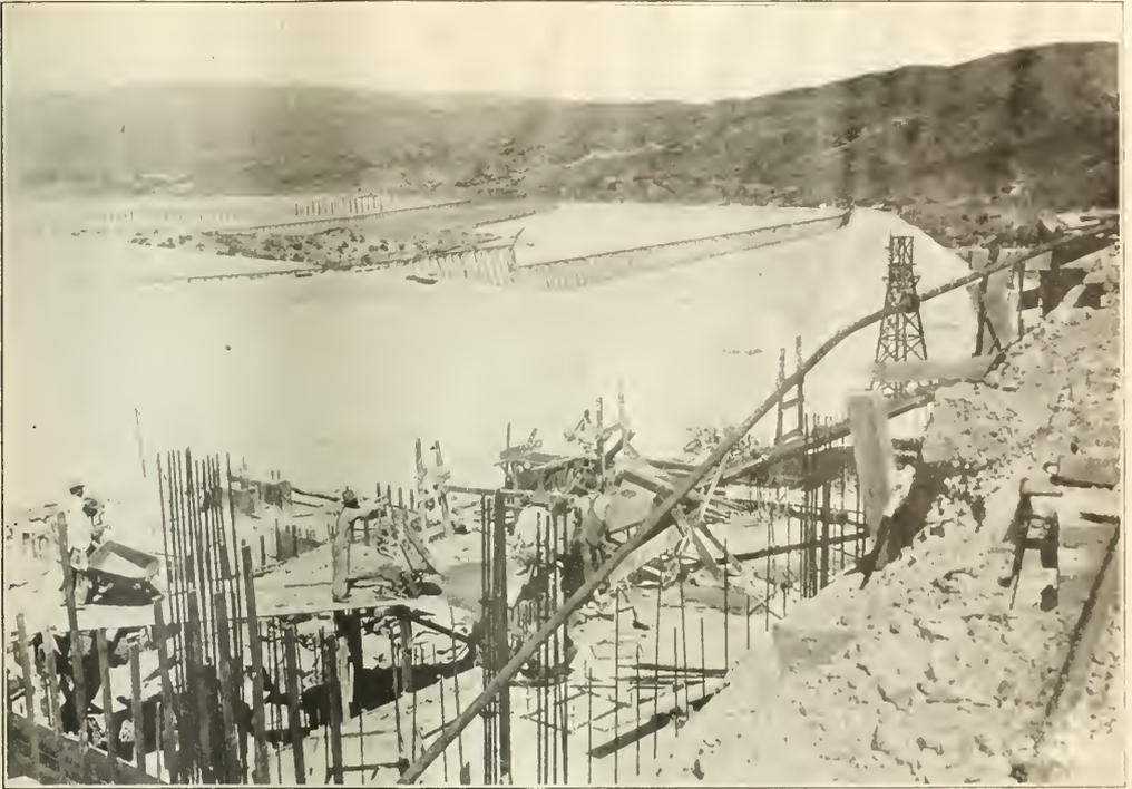
NEW CONSTRUCTION BY MIAMI COPPER CO. FOUNDATIONS FOR ORE CRUSHER PLANT AT NEW SHAFT
