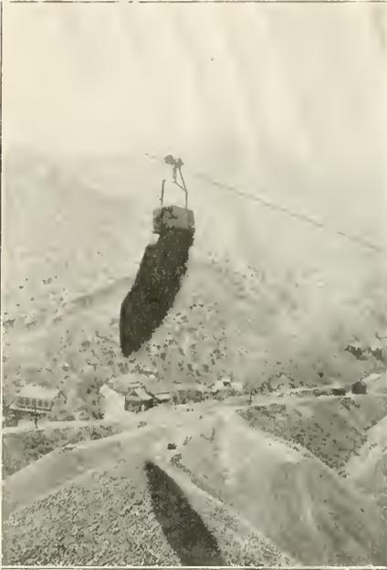
NEW IDRIA QUICKSILVER MINING CO., IN CALIFORNIA, DELIVERS RED HOT CALCINES TO DUMP BY AERIAL TRAMWAY
