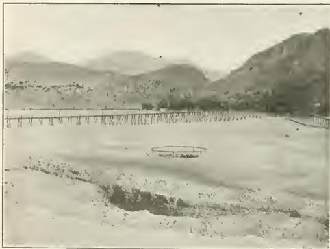
SOUTH CLIFTON SLIME TAILING POND, SHOWING PRELIMINARY SAMPLE CUT IN FOREGROUND AND TEST PIT IMMEDIATELY BEYOND
