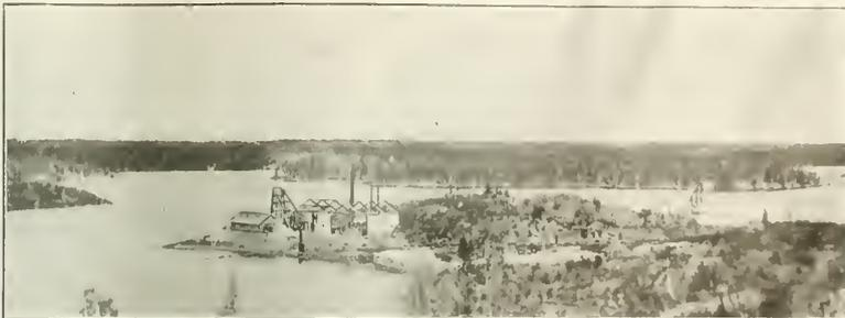
GENERAL VIEW OF FLIN FLON PROPERTY ON FLIN FLON LAKE, NORTHERN MANITOBA. SHOWING PLANT UNDER CONSTRUCTION AND HEADFRAMES AT TWO SHAFTS ABOUT 1,000 FT. APART. THE SMALL HILL BETWEEN SHAFTS IS A HORSE IN THE OREBODY
