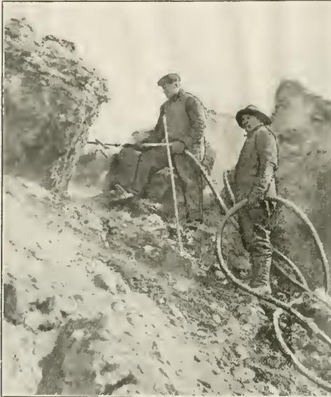
APPLICATION OF STEAM JET DRILLING FROZEN CHUNKS IN IRON MINING
