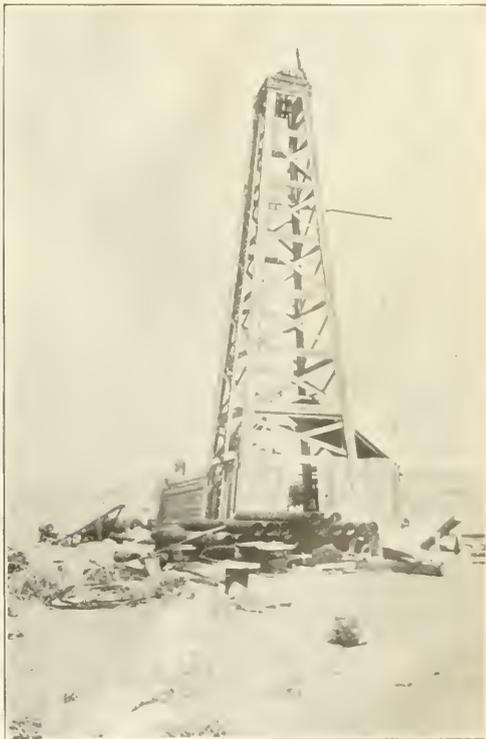
DERRICK USED WITH ROTARY RIG
