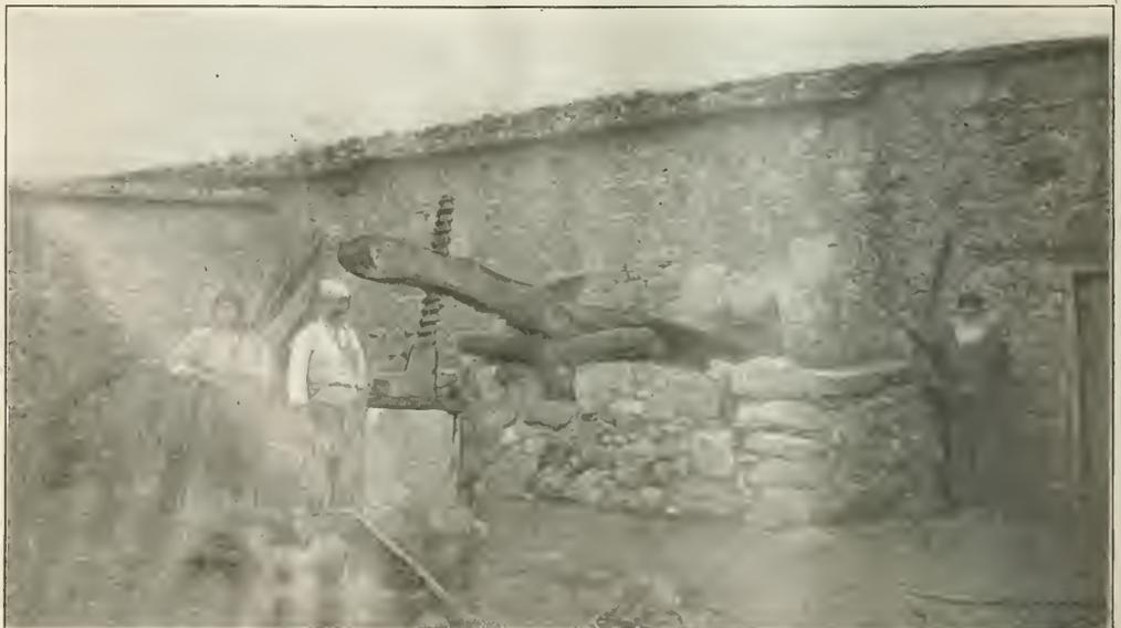
WINE PRESS AT KYKKO MONASTERY, POLEMI, CYPRUS. AT THE LEFT IS SHOWN THE WOODEN SCREW, BY MEANS OF WHICH THE NECESSARY PRESSURE IS OBTAINED
