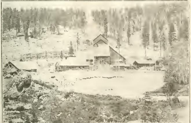
MILL AND TAILINGS POND AT ANACONDA COPPER MINING CO.'S WALKER MINE, PORTOLA, CAL. TRAMWAY TO UPPER MINE IS SEEN IN CENTER. SNOW SHED ON RIGHT BEYOND MILL LEADS TO LOWER TUNNEL.
