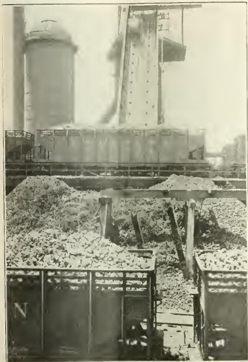
COKE AND IRON ORE AT SKIPWAY OF FURNACE
