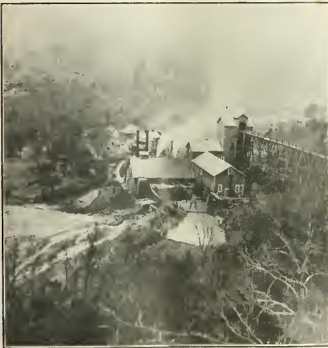
MODERN 200-TON CONCENTRATOR HANDLING ZINC CARBONATE ORE AT RUSH, IN NORTHERN ARKANSAS
