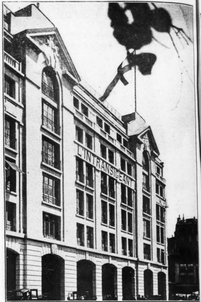
In the heart of busiest Paris, L'Intransigeant has located its new building, with six stories above the street level and three below. Near the upper left corner is shown a pediment which symbolizes news-gathering, the sculptor using the figures of the telephone operator, reporter and stenographer. The corresponding pediment shows in bas-relief the news-printing group—the compositor, proof-reader and pressman. At the lower left appears the main entrance, a large view of which is printed below.
