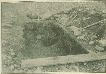
Photo No. 31. A deeper hole for the siphon
