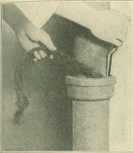
Photo No. 36. Packing oakum in joint
