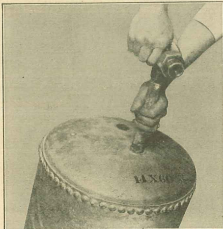
Photo No. 16. Dropping cold water pipe into boiler
