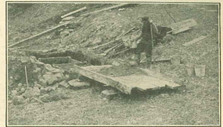
Photo No. 33. Ready to finish the concrete work
