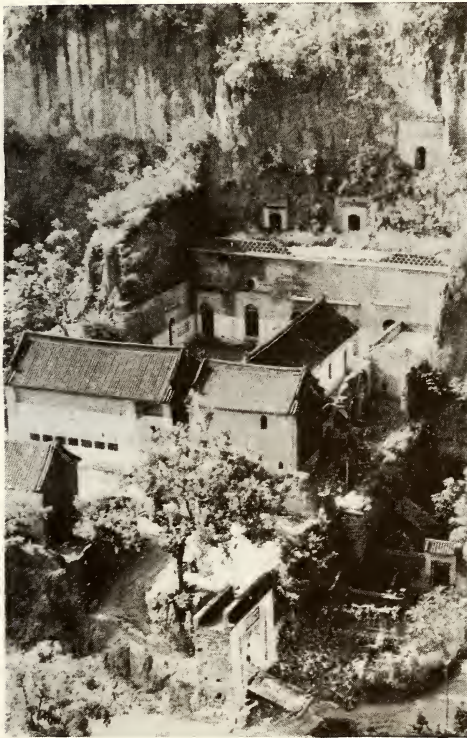
Figure 11: Hillside town development in China (a) Plans and sectional perspective (b) Hillside (elevational) dwelling known as a 'dragon cave' (Kakiuchi and Noguchi, 1985).
