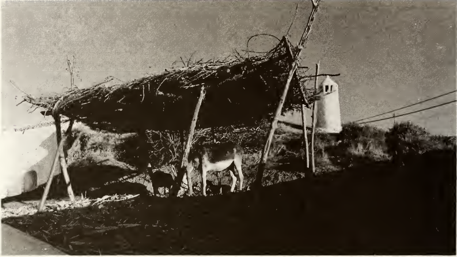
Figure 12: An earth-covered dwelling in the Spanish underground town of Guadix
