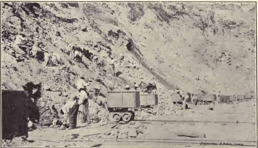
FIG. 35.—Openpit mining at Puertocitos.
