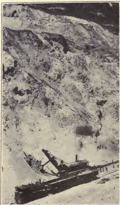
Fig. 30.—Shoveling 230-ft. bank, Utah Copper mine.
