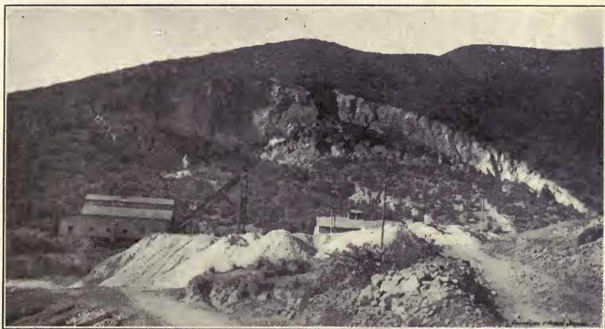
FIG. 103.—Caved ground, Veta Grande mine.
