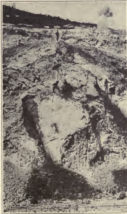
FIG. 31.—Trimming bank, Utah Copper mine.
