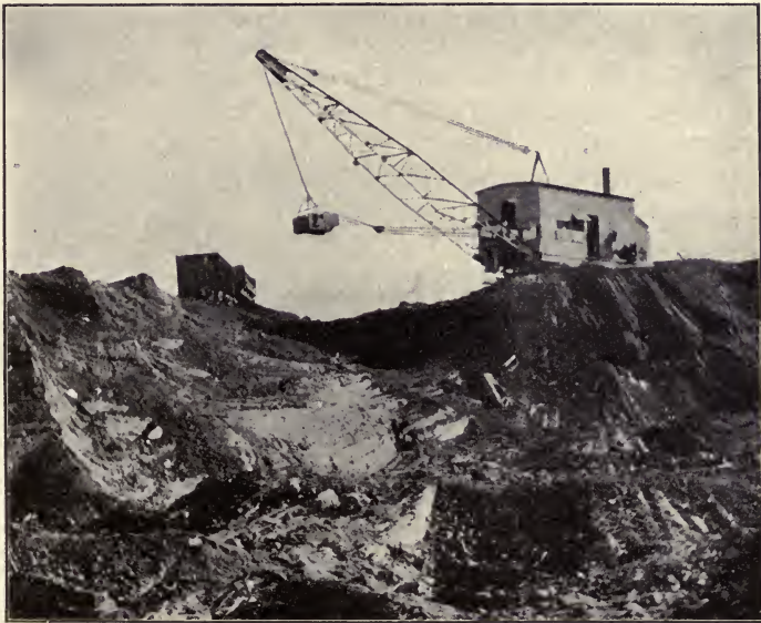
FIG. 25.—Drag-line excavator at Mayari, Cuba.
