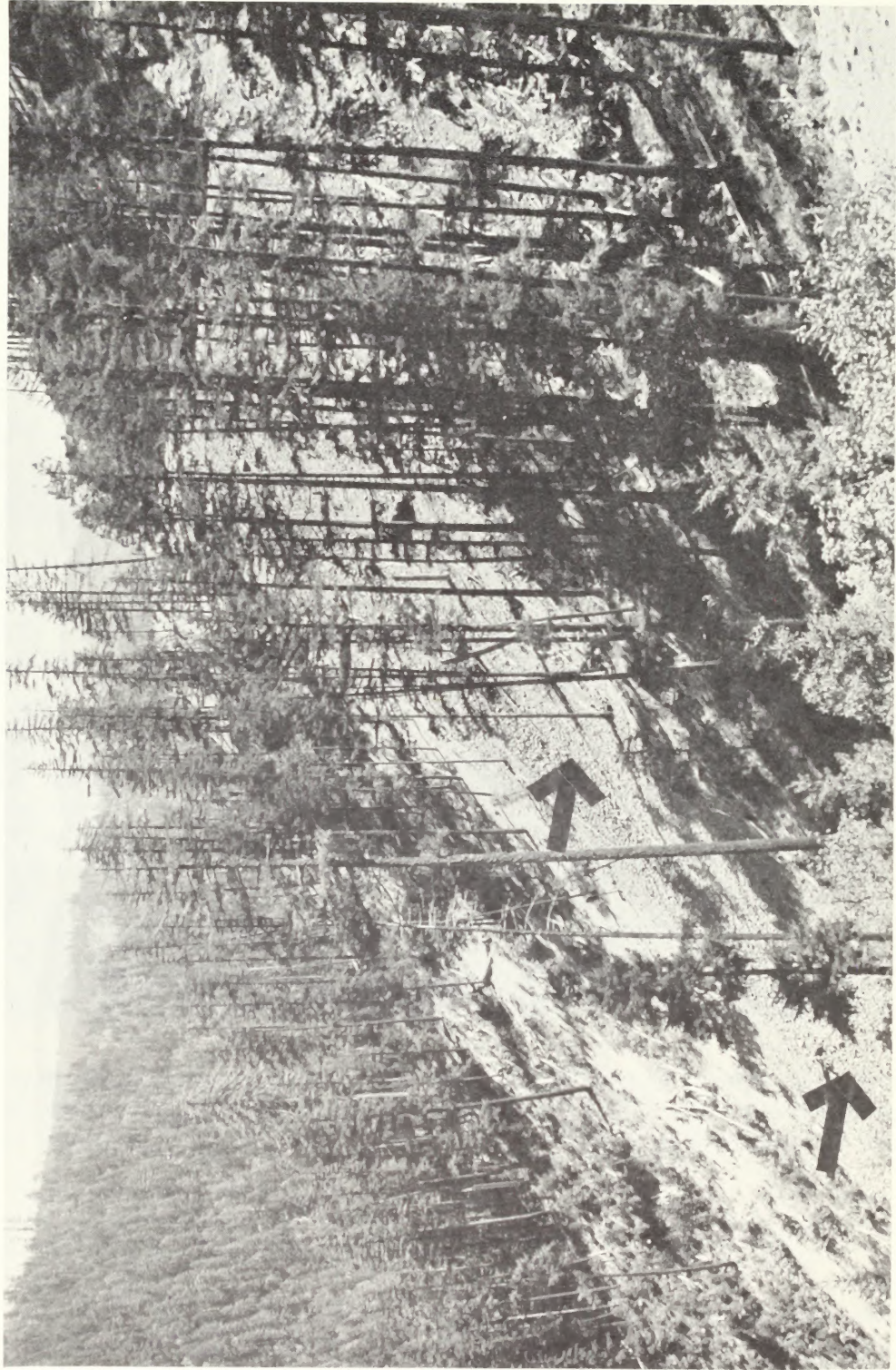
Figure 9. Very stony side-cast material on steep terrain extends far downslope reducing the productive land base.
