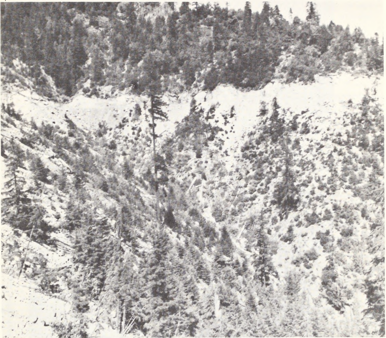
Figure 8. Roads on steep terrain usually result in deep cuts into the rock substratum. Side-cast material with high rock fragment content will not become revegetated.
