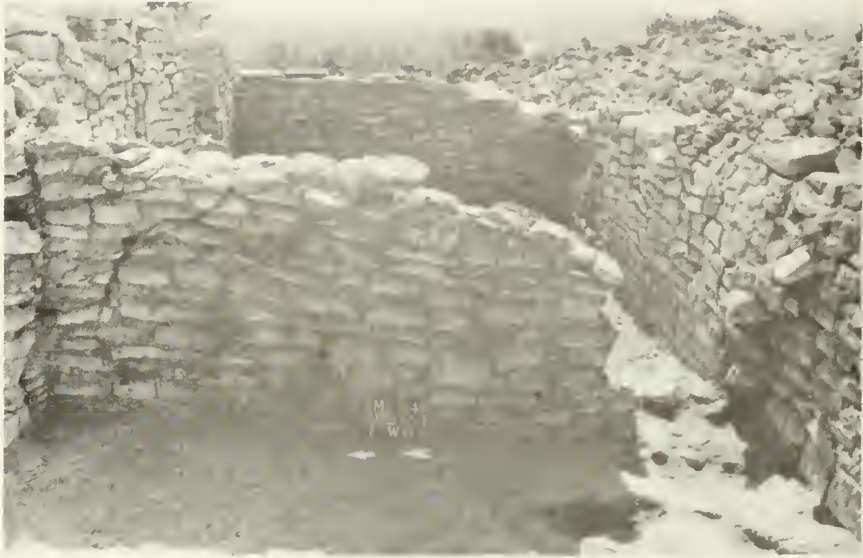
Figure 52: North wall of Room 20 showing the T-shaped door which opens to Room 10.
