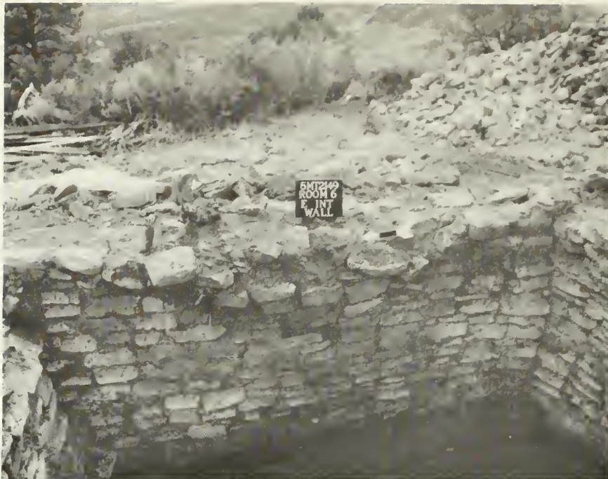
Figure 8: The east wall of Room 6 showing the Style 2 masonry.
