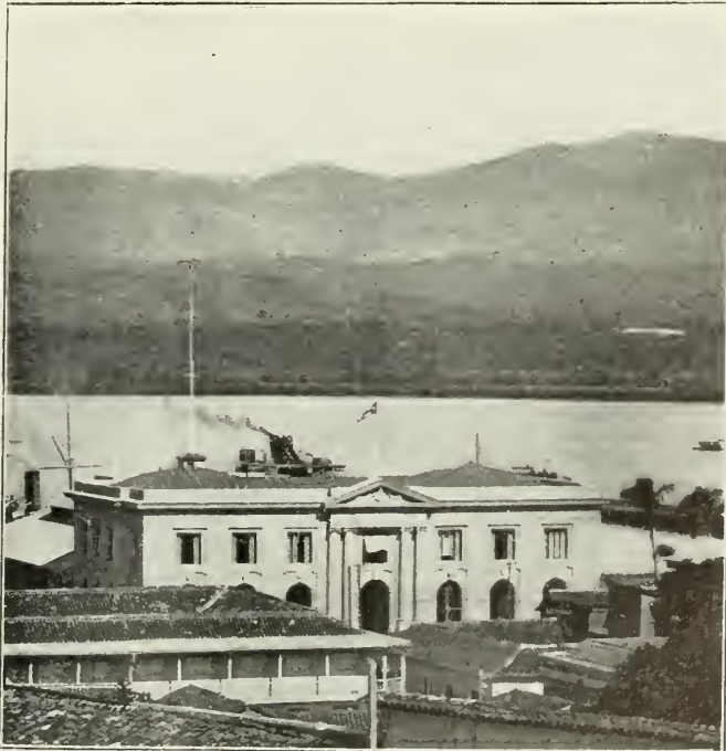
View of the new custom house at Santiago, but recently finished. It is in danger of collapse through faulty construction, say engineers.
