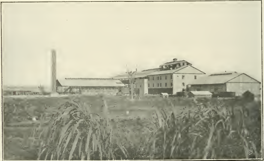
The new sugar mill of the Cuba Company at Jobabo, Oriente Province. It is the newest in the sugar group and only began grinding in February.
