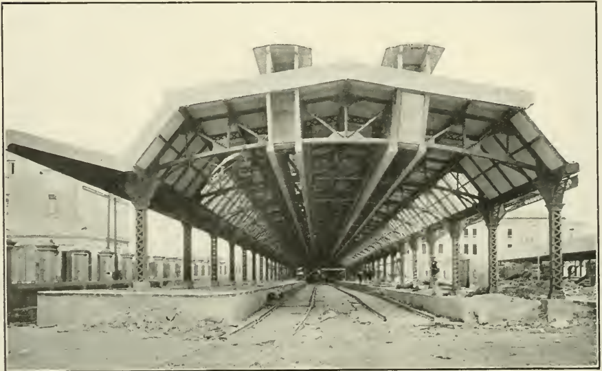
Interior view of the new train shed of the Havana Terminal Co. in the Arsenal Yard.
