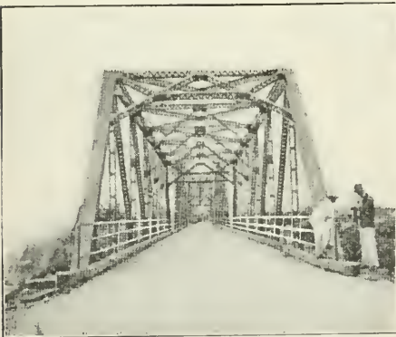
Steel bridge recently built over the Zaza River near Sancti Spiritus, Santa Clara Province. The length of the bridge is 228 meters.
