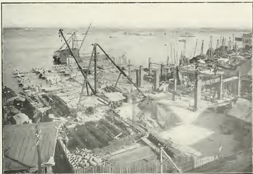
Illustration No. 1, taken in January. A view of the concrete piers in Havana Harbor now being built by the Port of Havana Docks Company. See details on this page.
