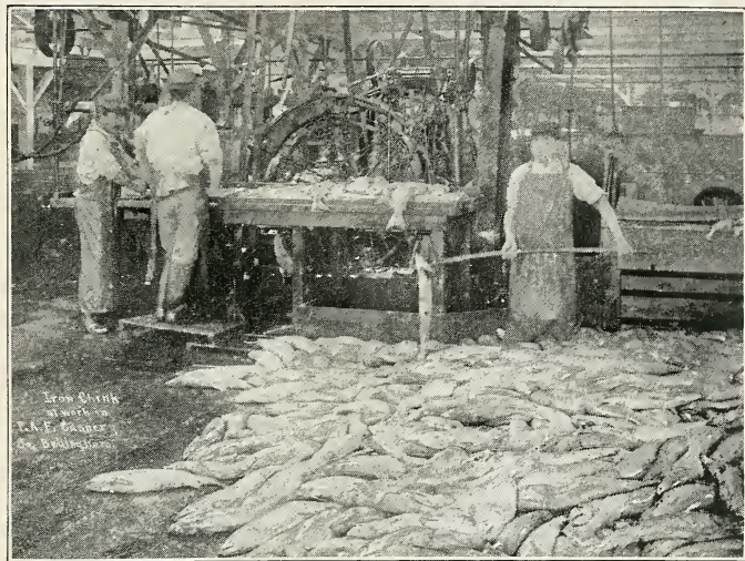
Feeding salmon to the "Iron Chink." This machine, which has largely displaced the Chinaman in the canneries, can cut and clean fifty fish in a minute
