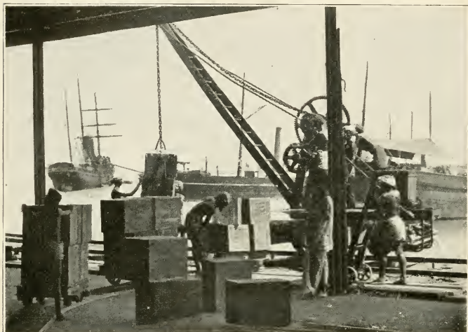
Loading tea at the dock with the aid of a hand derrick
