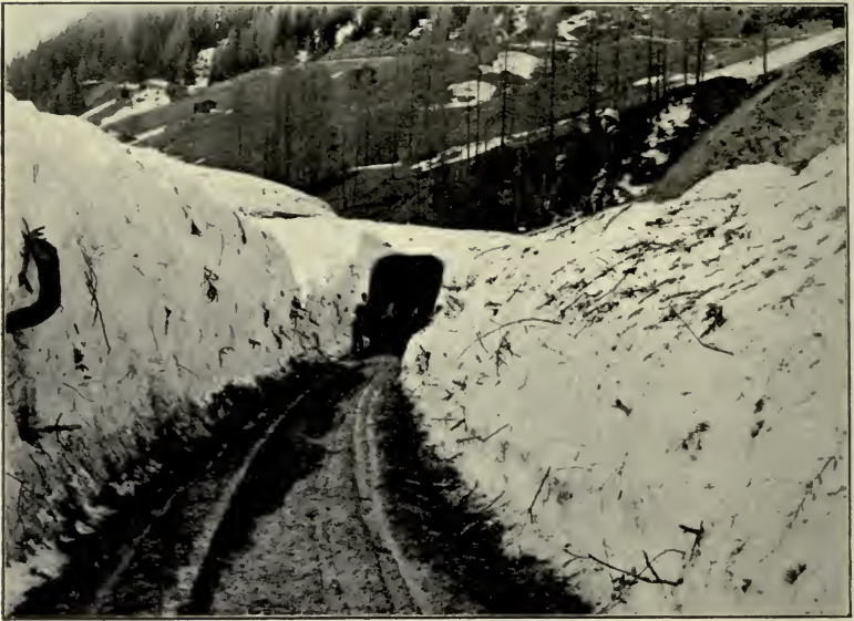
A TUNNEL 300 FEET LONG THROUGH AN AVALANCHE. Tree trunks, etc., can be seen embedded in it.
