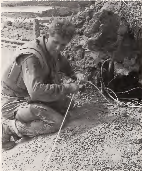
Photo from the Abel Collection Marine engineer LCpl Jerry Kanone runs a detonating cord from a charge placed inside an enemy bunker that can be seen at the right of the picture.
