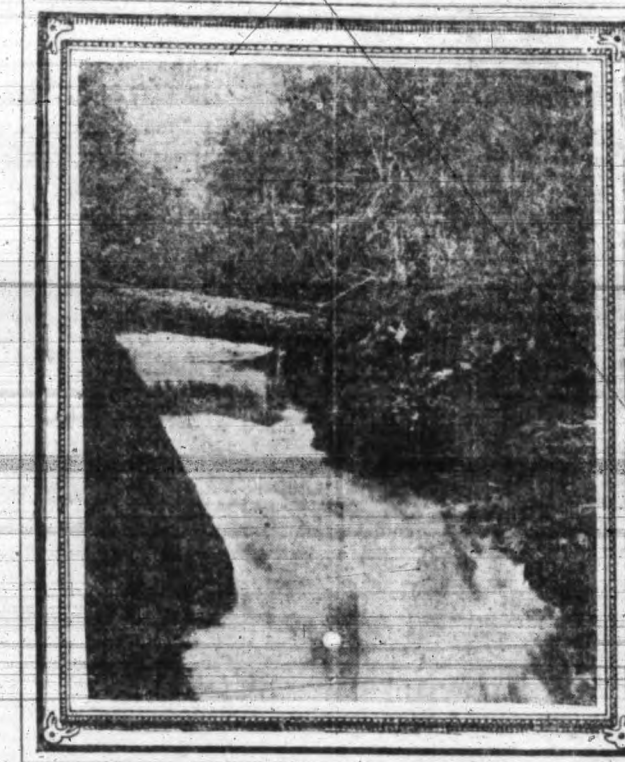
WEIR NO. 1 IN THE HIGHLAND DISTRICT. Photo Taken When Gauge Was Recording a Flow of Over Sixty-Five Millions per Twenty-Four Hours.
