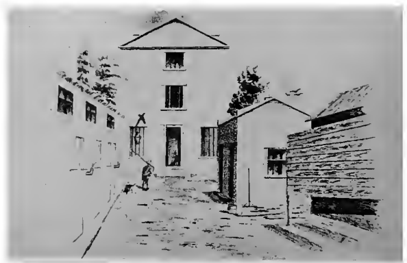
REAR OF JAIL AND YARD
