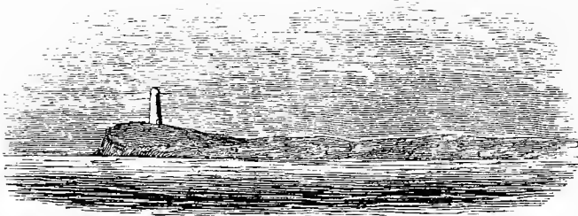
View of Montauk Point, Long Island.
