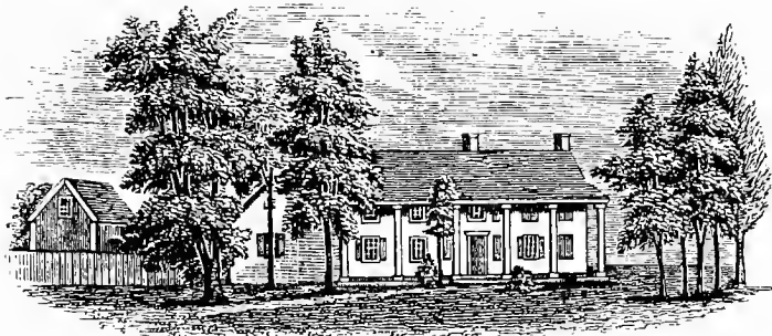
Schuyler mansion-house, Schuylerville.
