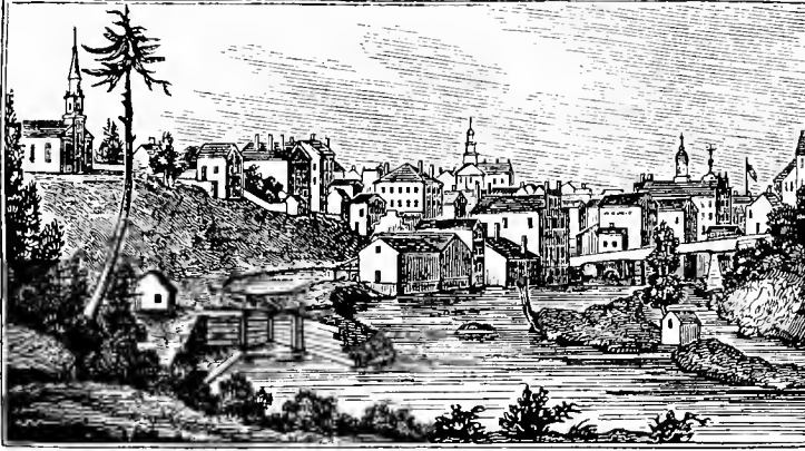
East view of Seneca Falls village.
