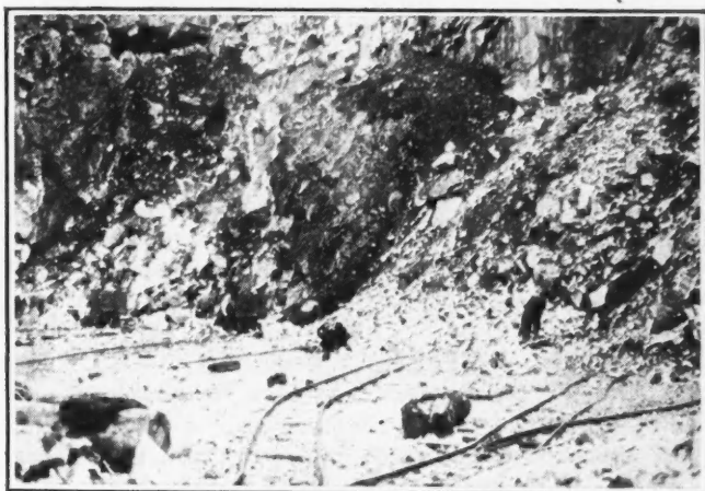
Small-scale limestone quarrying, showing track layout for hand tramping or horse haulage
