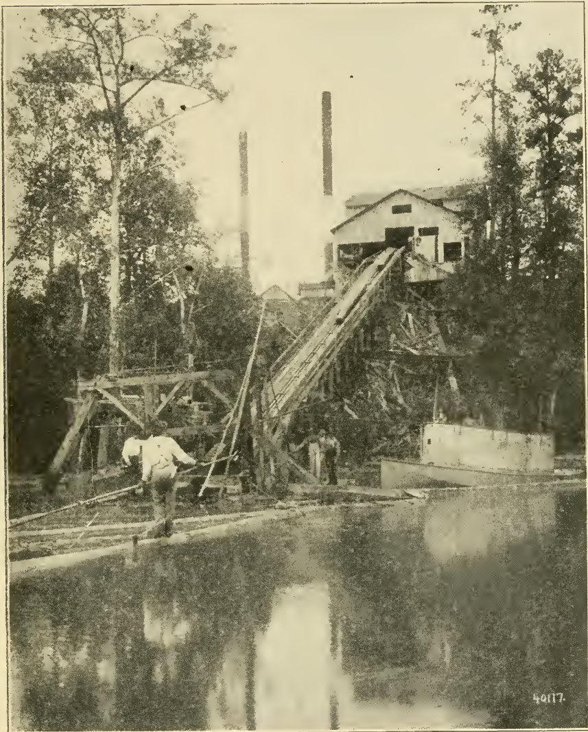
FIG. 213. LOG SLIDE AT A MILL IN SOUTHERN GEORGIA.
