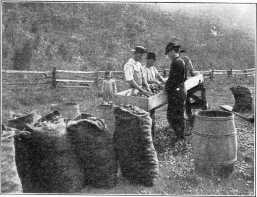
FIGURE 17.—Grading onions in the field by means of a screen
