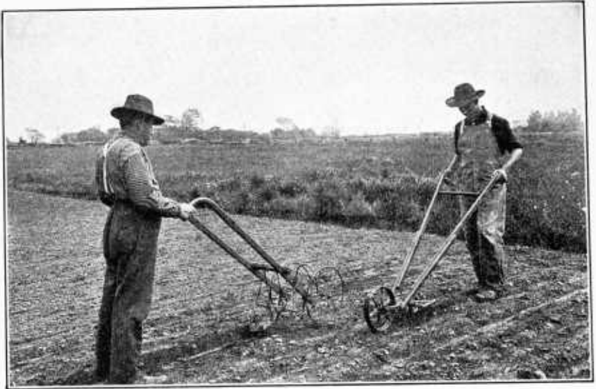
FIGURE 6.—Special wheel hoes for cultivating onions
