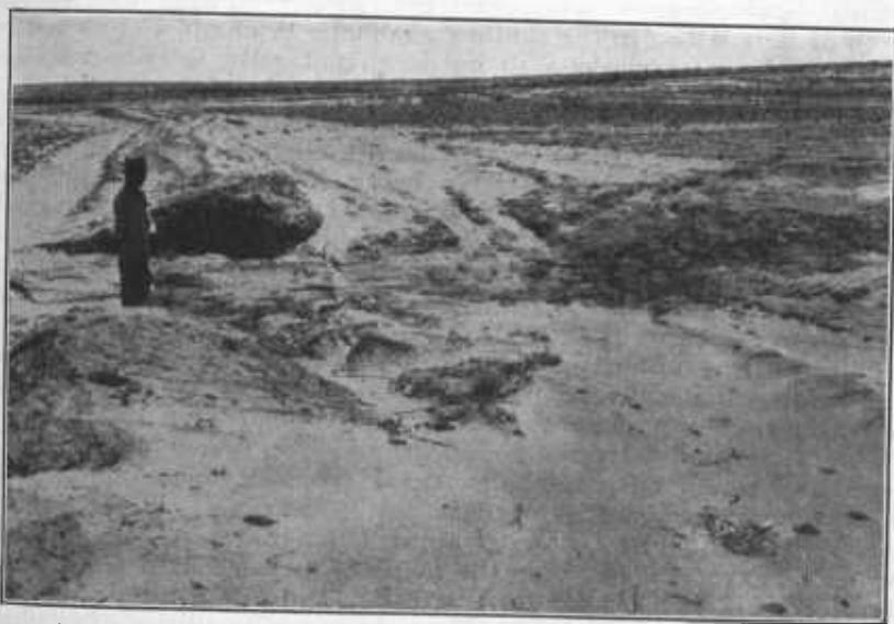
FIGURE 8.—Overtopping, caused by improper design, construction, or maintenance of terraces, damages both field and terrace.
