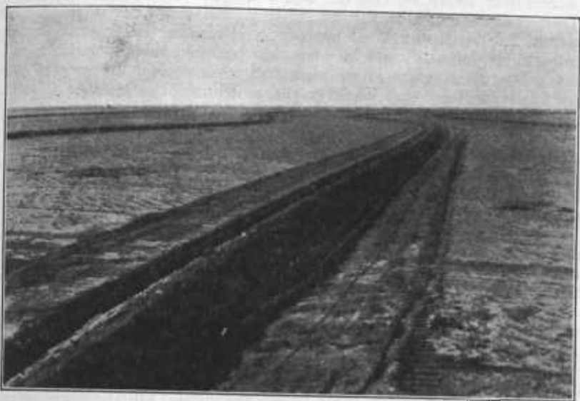
FIGURE 27.—Partly constructed terraces in the Great Plains, where slopes are relatively flat and uniform.
