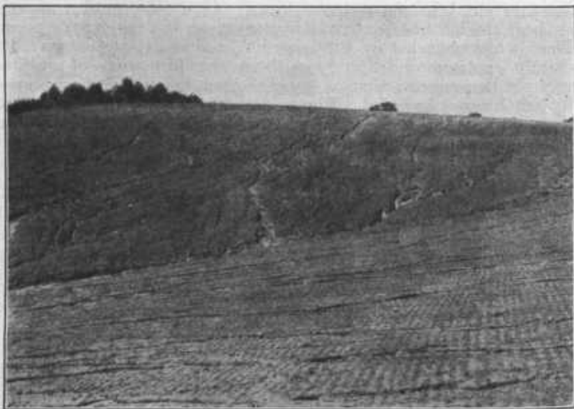
FIGURE 4.—Sheet erosion that has developed into the fingering or shoestring stage of gully erosion.
