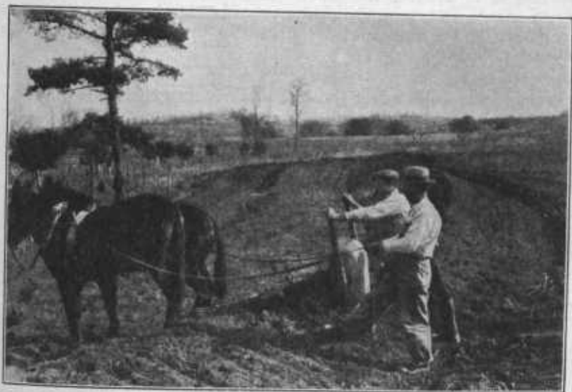
FIGURE 28.—Making use of a slip scraper and team to fill low places in a terrace ridge.
