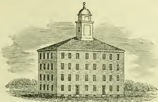
Collegiate building at Brockport.
