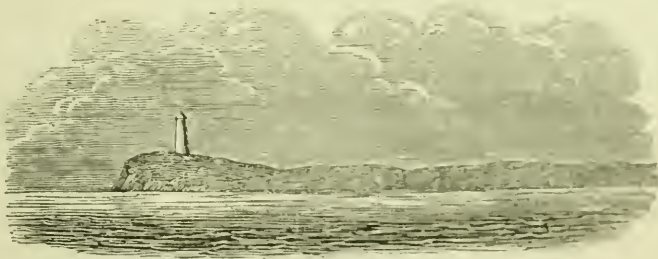
View of Montauk Point, Long Island.
