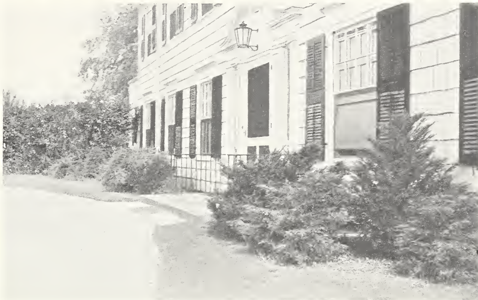
A good type of foundation planting, Japanese Yew and Juniper. Professor E. Gorton Davis of the School of Landscape Architecture, Cornell University has designed this for the late Robert E. Ahles, Westbury to show correct principles of foundation planting. It shows part of the foundation. It has horizontal, not vertical lines, harmonious foliage, not a conglomerate mixture. The plants will stay small, not quickly cover the windows.
