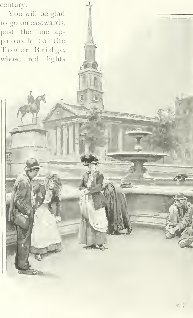
MORNING TOILET (TRAFALGAR SQUARE).
