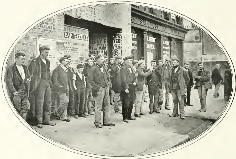
BUILDERS' MEN READY FOR WORK.
