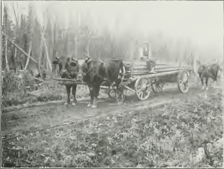
Road south of Heaslip.
