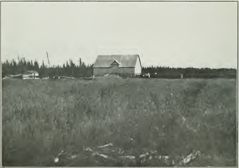
L. Bieleek's farm, Con. 6, Township of Lamarche, 3 miles west of Cochrane.
