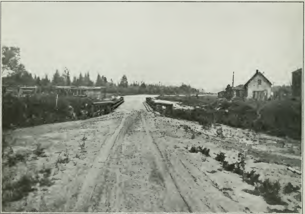
Part of the North Bay and Sturgeon Falls Trunk Road at Meadowside.
