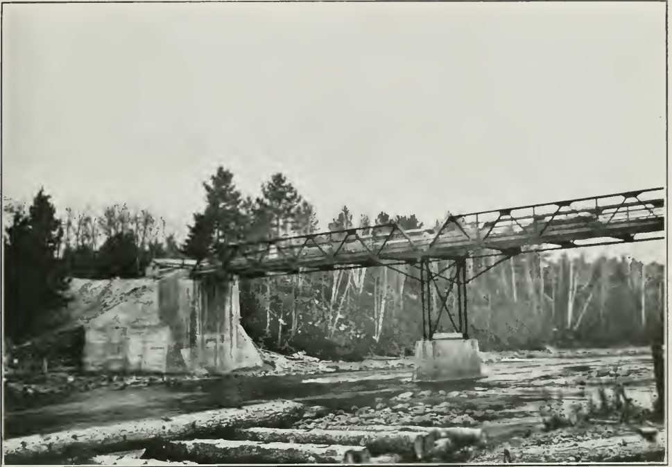
Iron Bridge across the Petawawa River on the Pembroke and Petawawa trunk road. length of bridge 180 feet, height above water 30 feet.
