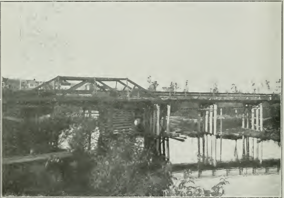
Bridge, 270 feet long, constructed in 1915 at the mouth of Bear Creek, near Elk Lake.
