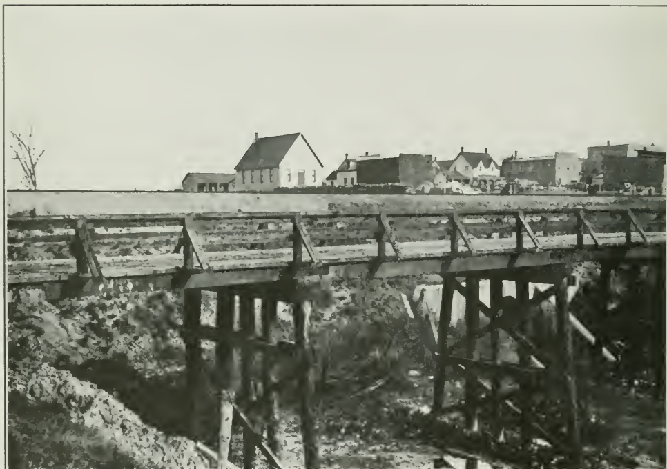
Bridge 175 feet long constructed at Warren on the C. P. R., 1915, on the trunk road from Sturgeon Falls to Sudbury.
